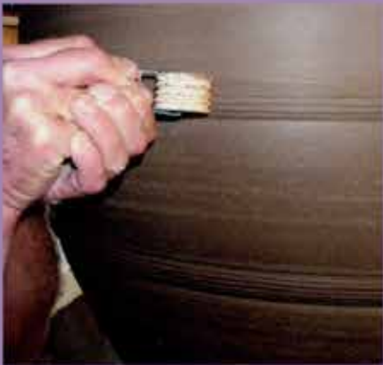
Applying surface detail with roller
